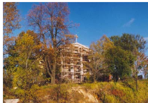
The Seminary under Construction – 1997
